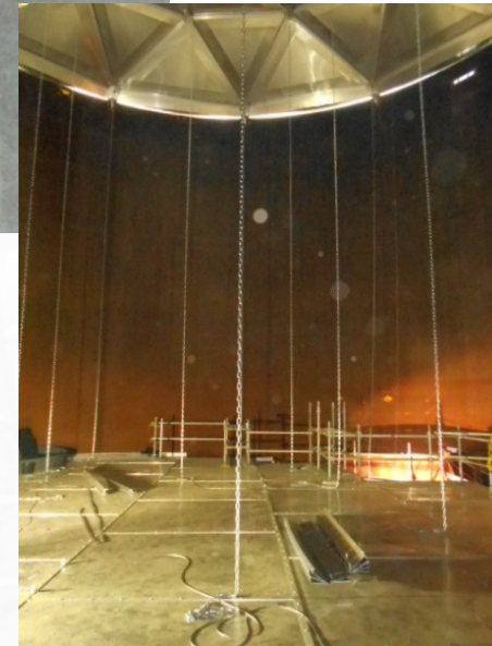
Cable / chain suspended
