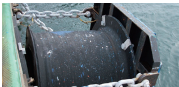
Insufficient bonding
