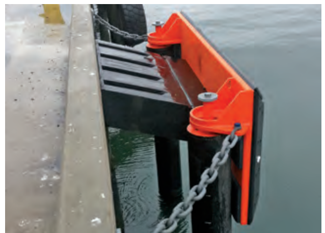
Pier 1 | North Kingstown, RI | USA
