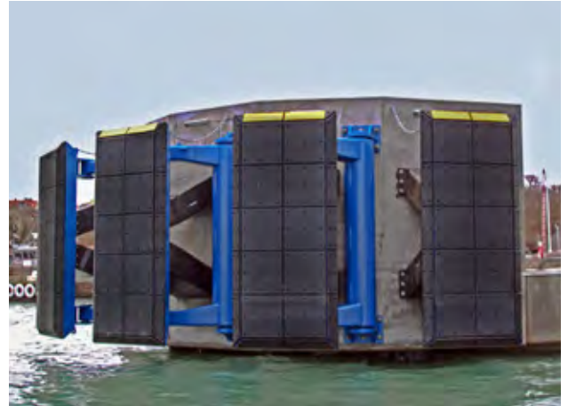
Ferry Terminal | Gotland Island | Sweden
