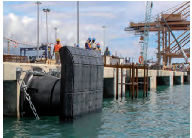
Mauritius Container Terminal | Port Louis | Mauritius
