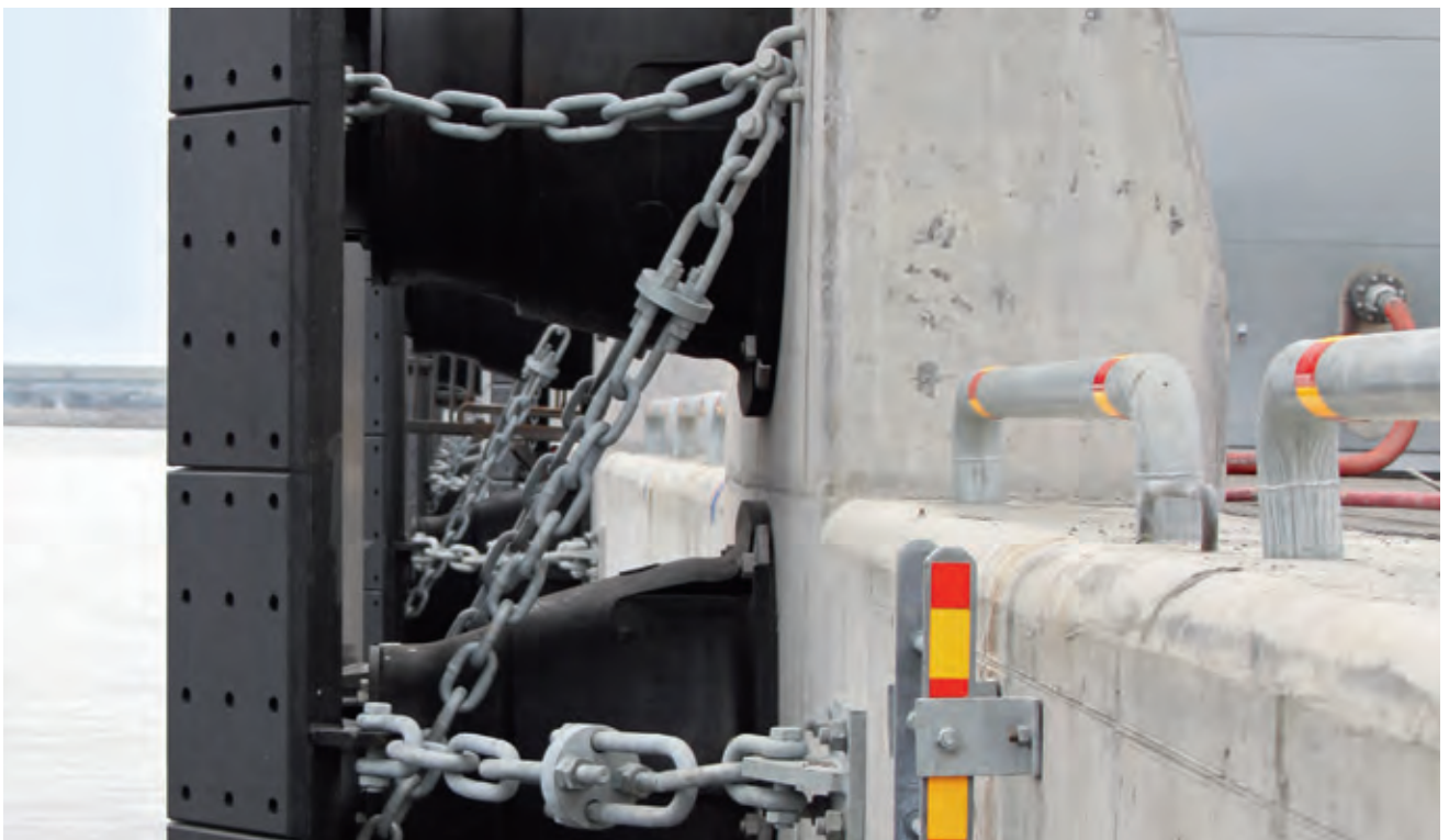
Restraint chain assemblies and brackets
