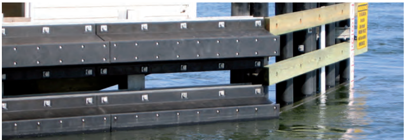
Margate Bridge | Margate City, NJ | USA
