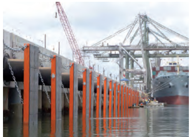
Barbour's Cut Container Terminal | Houston, TX | USA
