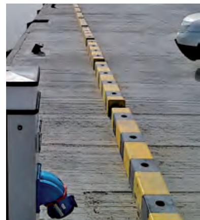
Southern Quay Wall | Simaisma | Qatar
