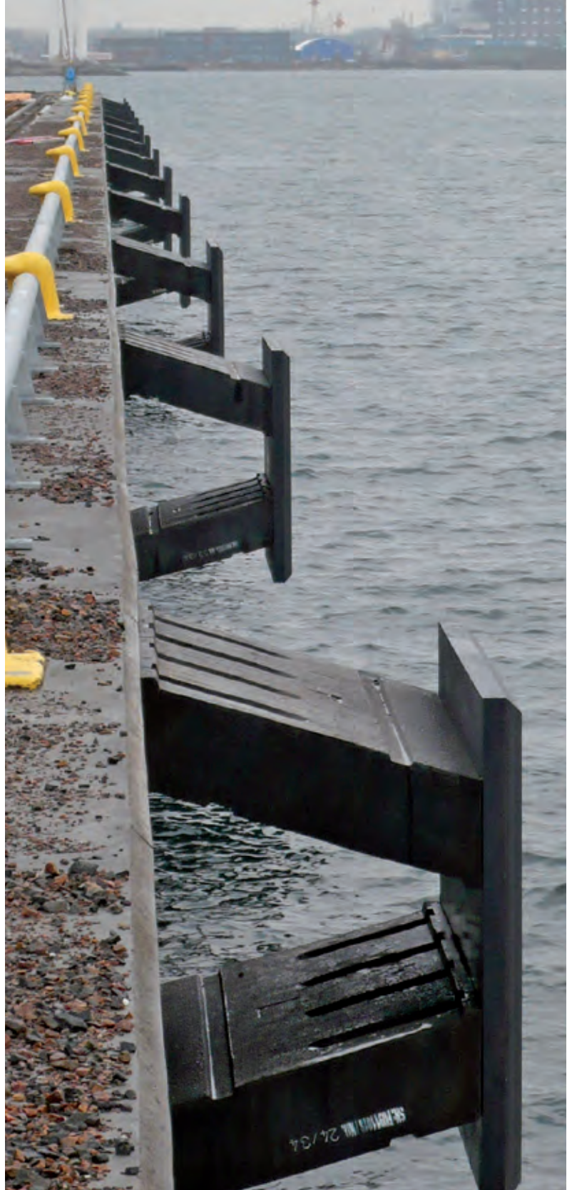
Ferry & RoRo Terminal | Malmö | Sweden
