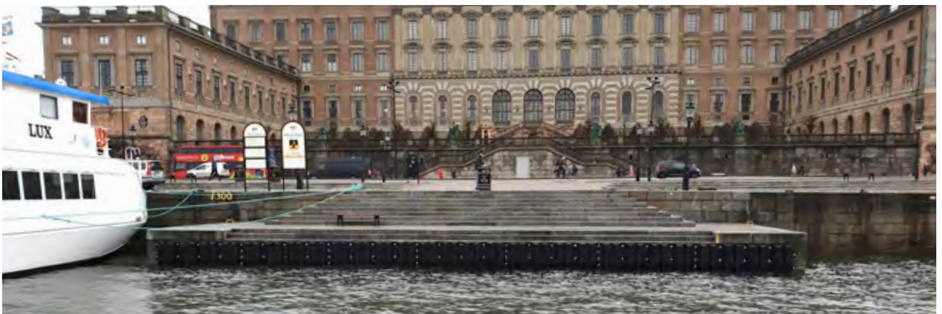
Logårdstrappan | Stockholm | Sweden
