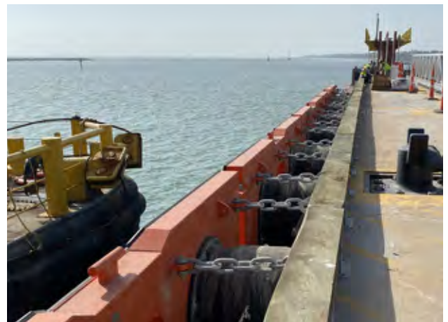
RoRo Facility | Portland, TX | USA
