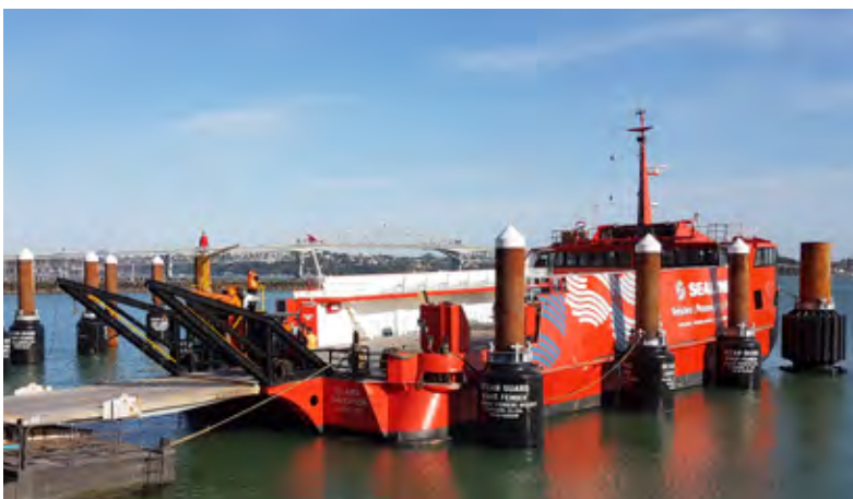
SeaLink Terminal | Auckland | New Zealand
