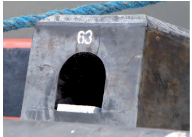
Offshorebasis Cuxhaven LP 8 | Germany
