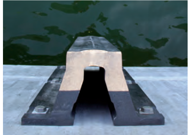
Ferry & RoRo Terminal | Kapellskär | Sweden
