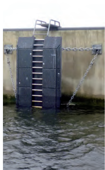
Maasvlakte II | Rotterdam | The Netherlands
