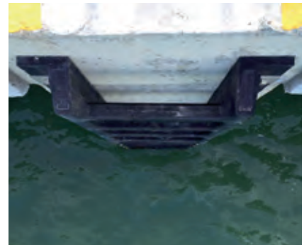
Feed Solid Product Jetty | Johor | Malaysia
