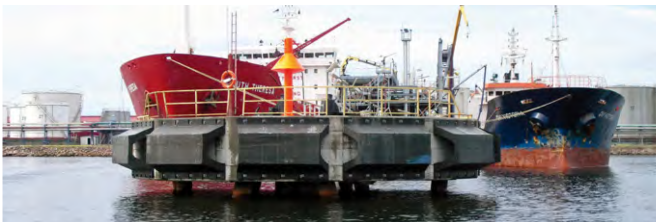
Oil Terminal | Muuga | Estonia
