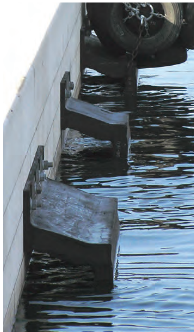
Passenger Terminal | Rijeka | Croatia
