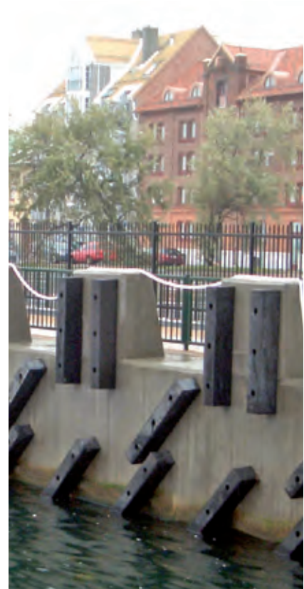
Ferry Terminal | Landskrona | Sweden
